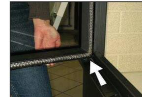
2. Then swing the door inwards and set the lower pin into the lower fixture. To ensure the hexagonal socket can slide into the fixture, move the door a little (swivel the door).
