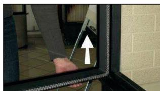
4. In this position, pull the door a little forward at the bottom.
