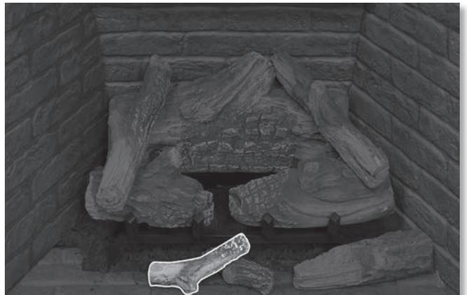
Figure 85: Log Set Installation - Step 8
